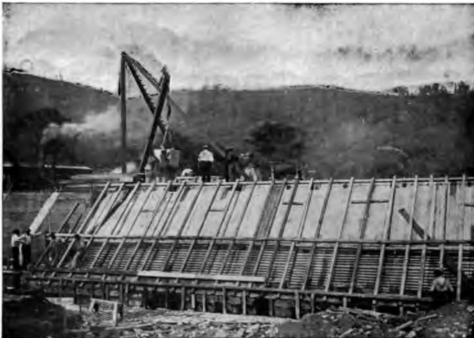
JUNIATA DAM. CONSTRUCTING DECK OF REINFORCED CONCRETE.
