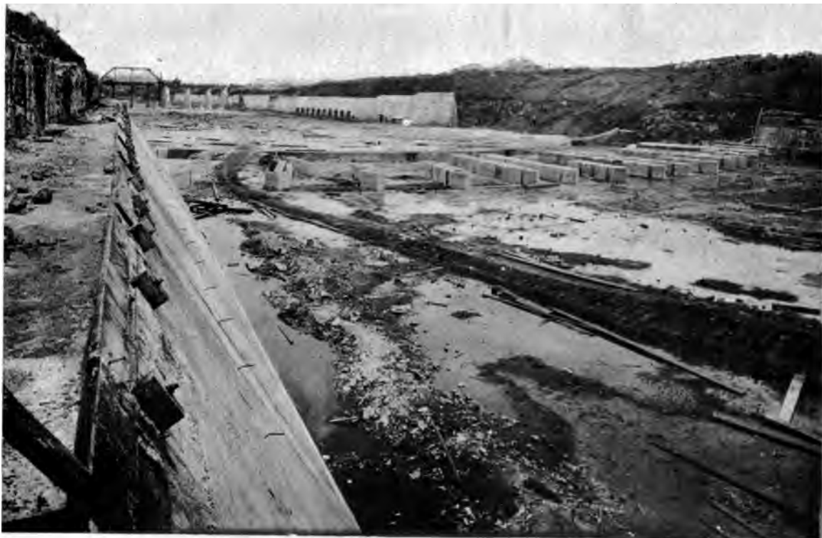
SPILLWAY OF THE GATUN DAM, LOOKING NORTH. Foundations for Valve and Cofferdam Piers in Foreground. (April, 1910.)
