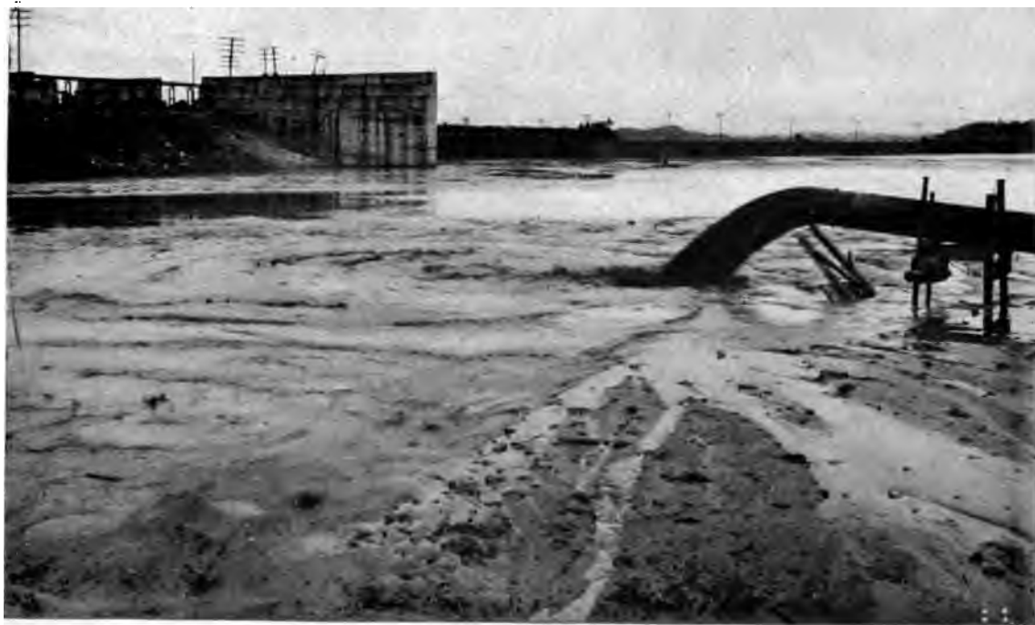
HYDRAULIC FILL OF THE GATUN DAM, EAST OF SPILLWAY. Suction Dredge Lift, 63 feet; Length of Pipe, 4300 feet. (August, 1910.)
