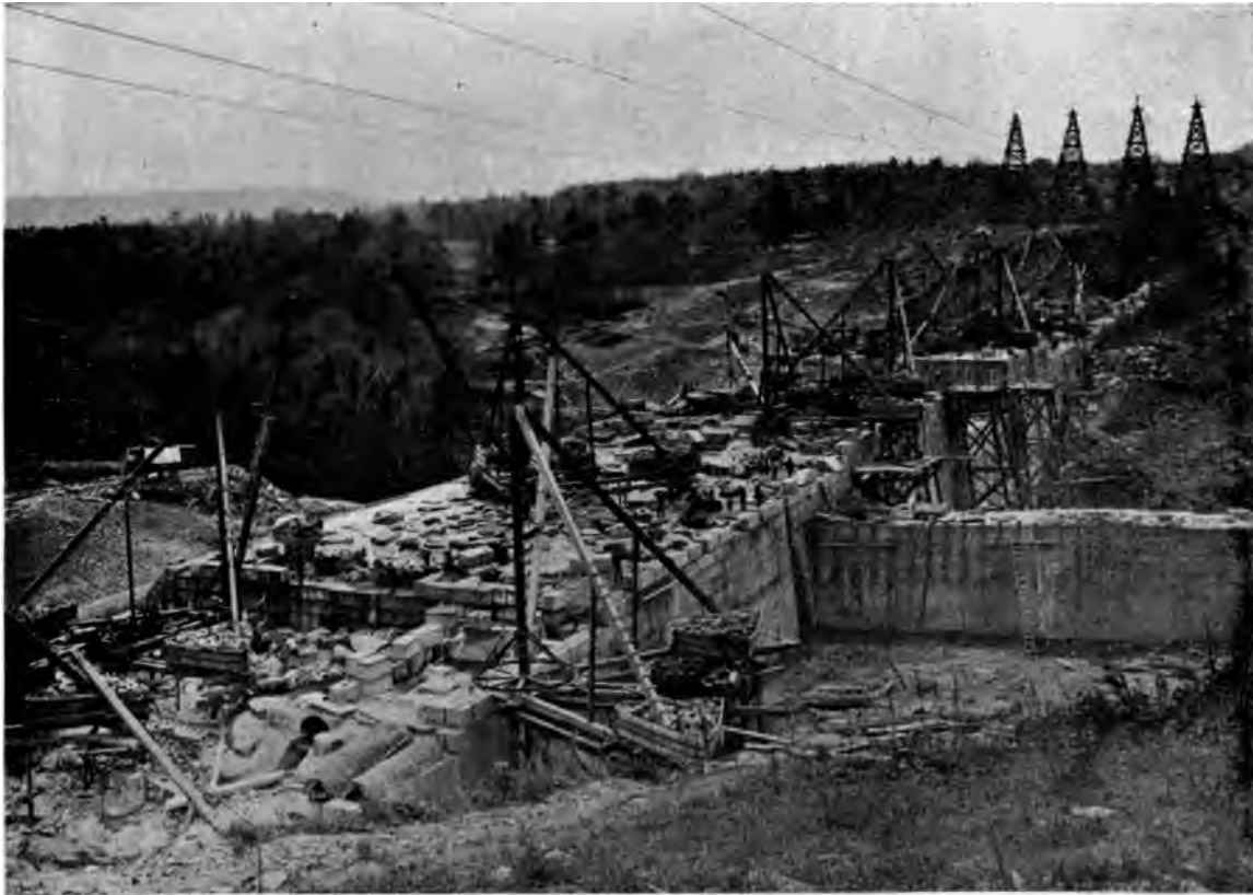
OLIVE BRIDGE DAM. UP-STREAM FACE. The wall at right angles to the dam is a temporary construction.
