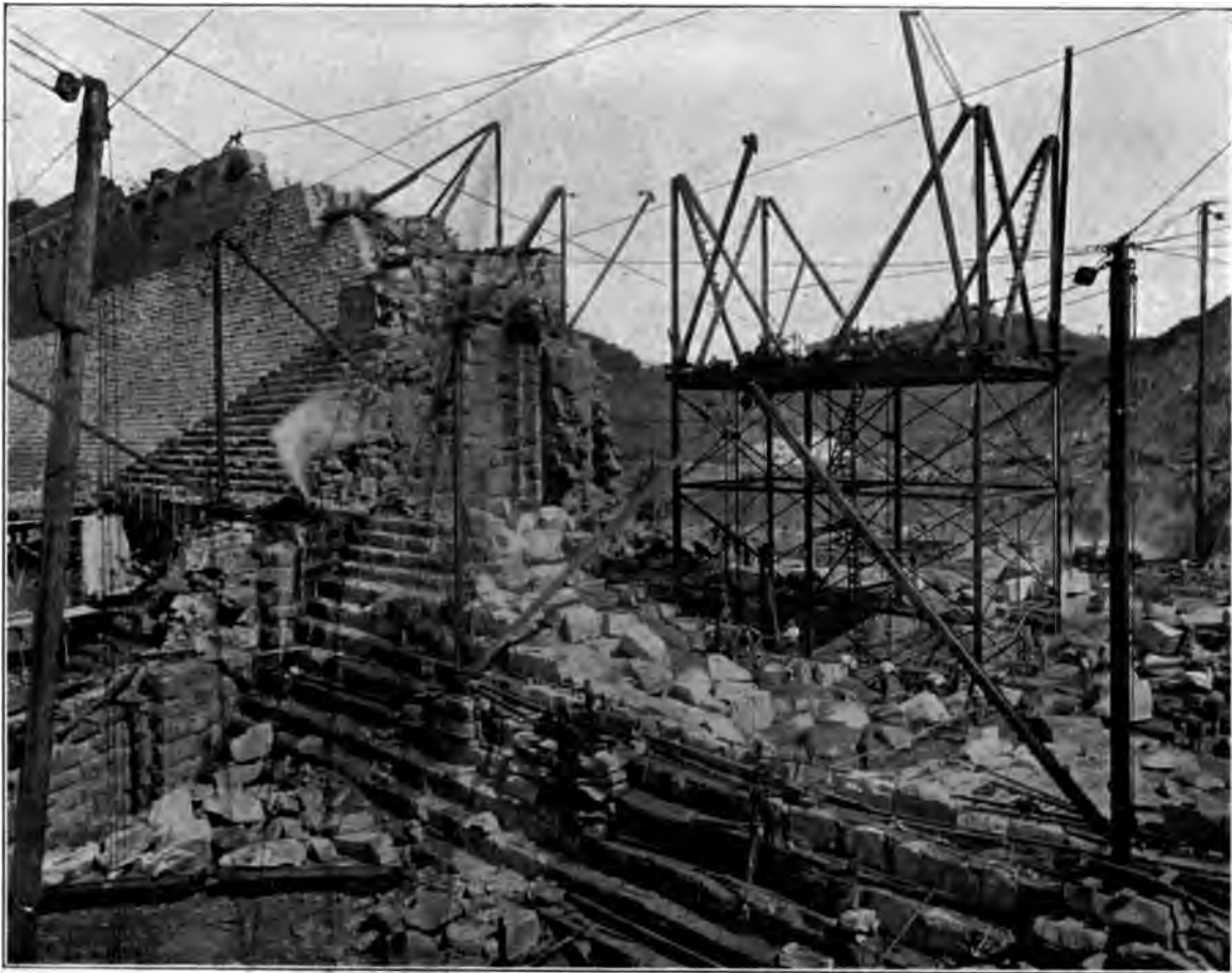
NEW CROTON DAM. DERRICK PLATFORM.
