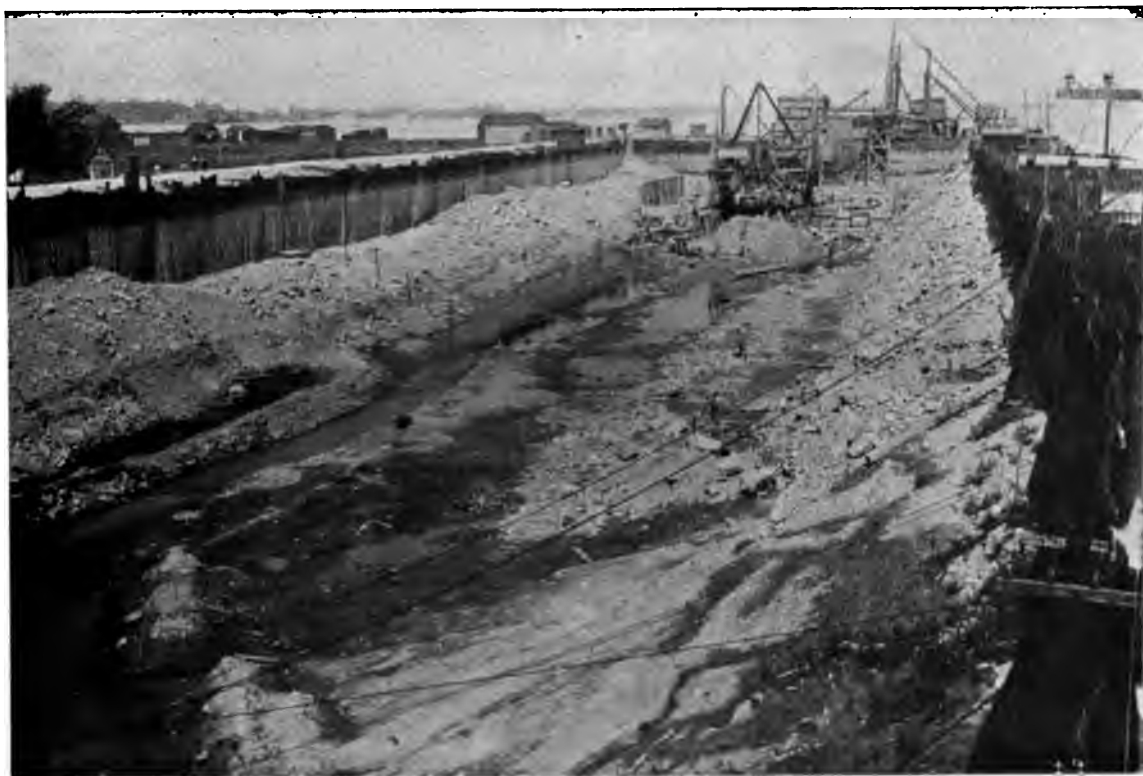
EXCAVATING IN COFFER-DAM IN BLACK ROCK HARBOR.
