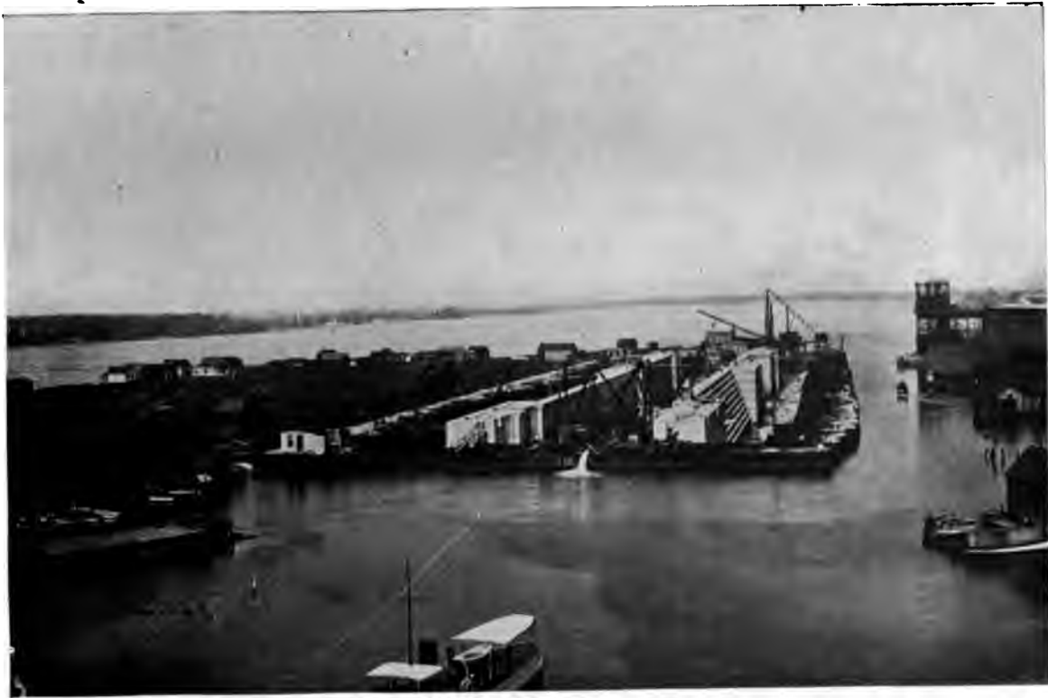
COFFER-DAM FOR CANAL-LOCK IN BLACK ROCK HARBOR, BUFFALO, N. Y.
