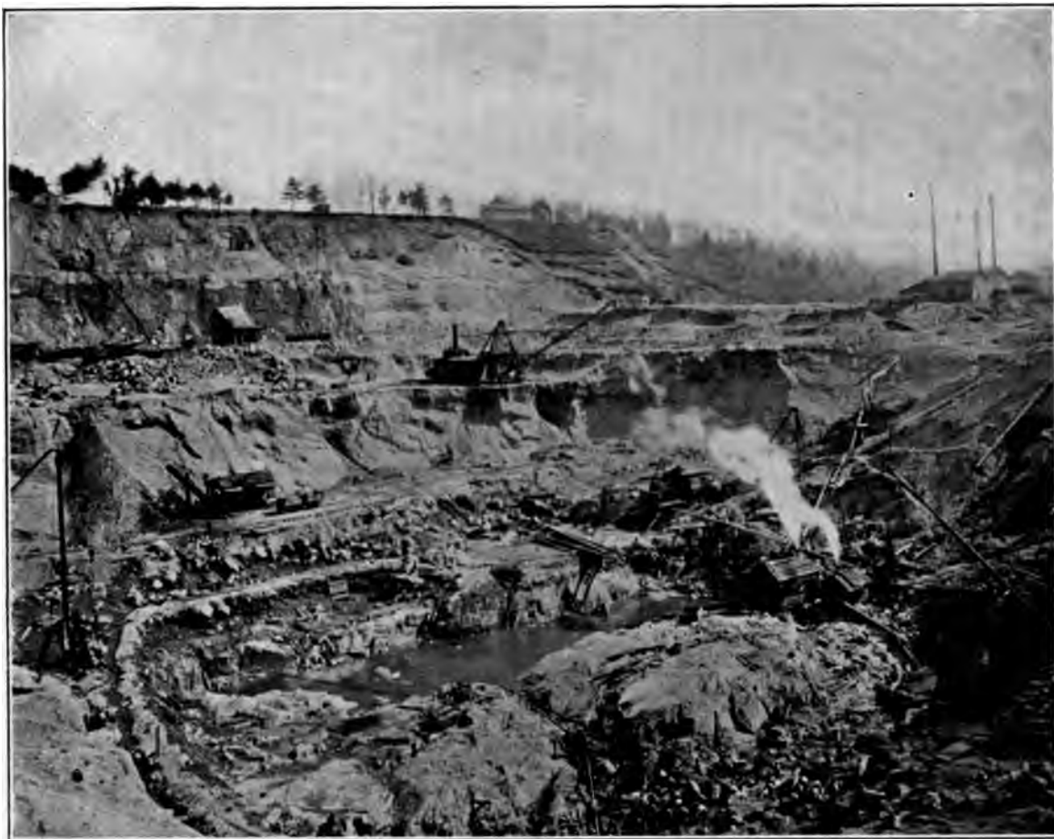
NEW CROTON DAM. EXCAVATING FOR FOUNDATION.
