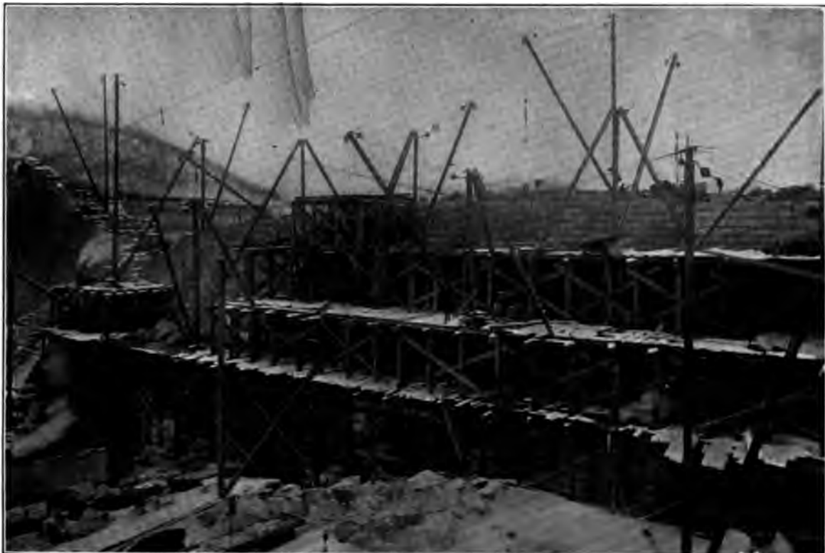
NEW CROTON DAM. TRESTLE ON DOWN-STREAM FACE.
