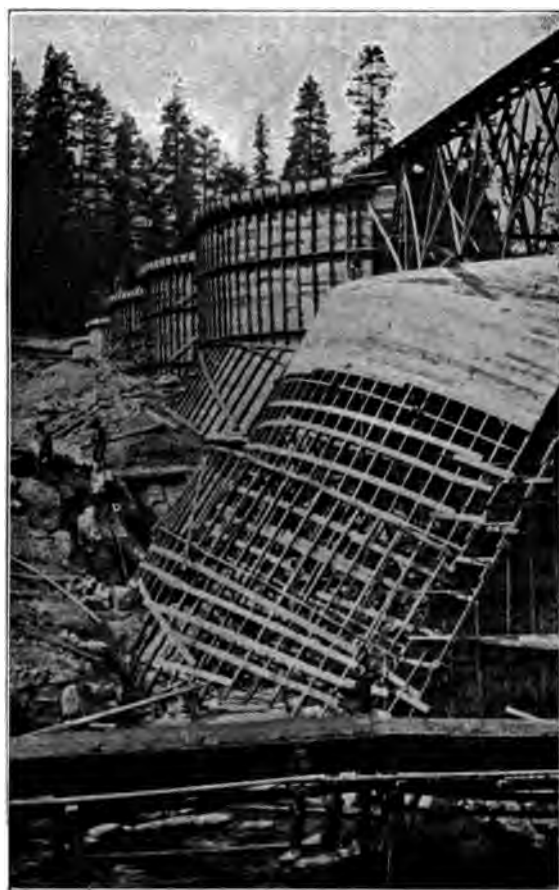
FIG. 179.—DETAIL OF ARCH FORM CONSTRUCTION.
