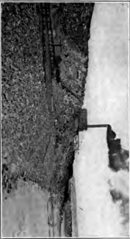
FIG. 3.—Rip-rap on Up-stream Face
