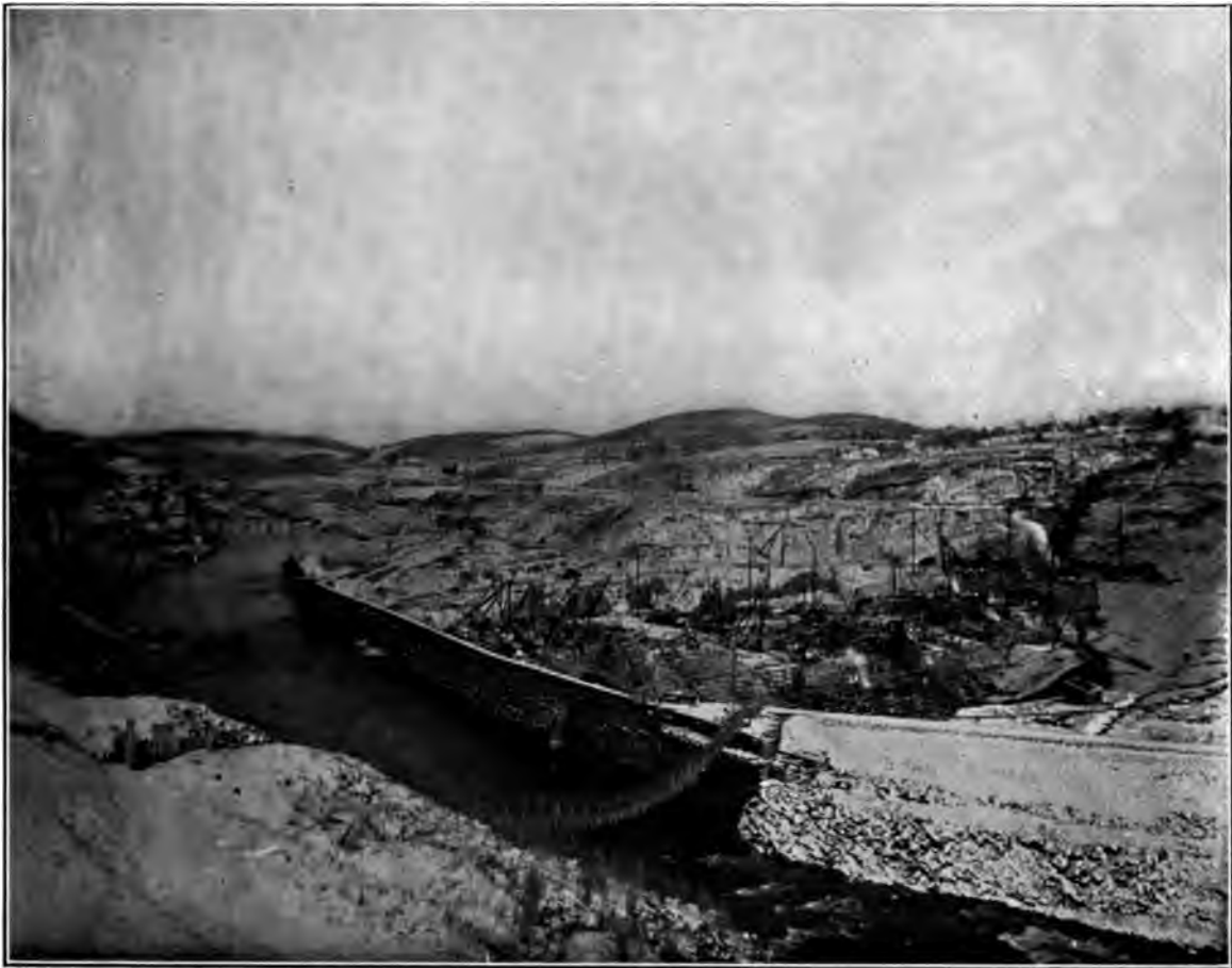
NEW CROTON DAM. TEMPORARY CHANNEL.
