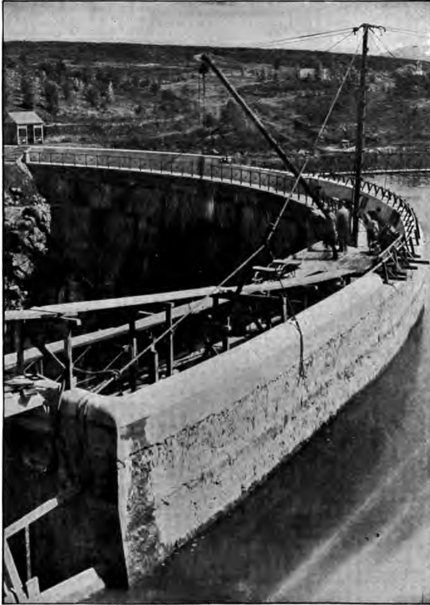
SWEETWATER DAM.—INCREASING THE HEIGHT OF THE PARAPET. (From "Eighteenth Annual Report U. S. Geological Survey.")
